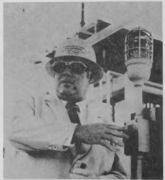
Lt. Governor of Aruba O. S. Henriquez turns switch for the official startup of the hydrodesulfurization units.
